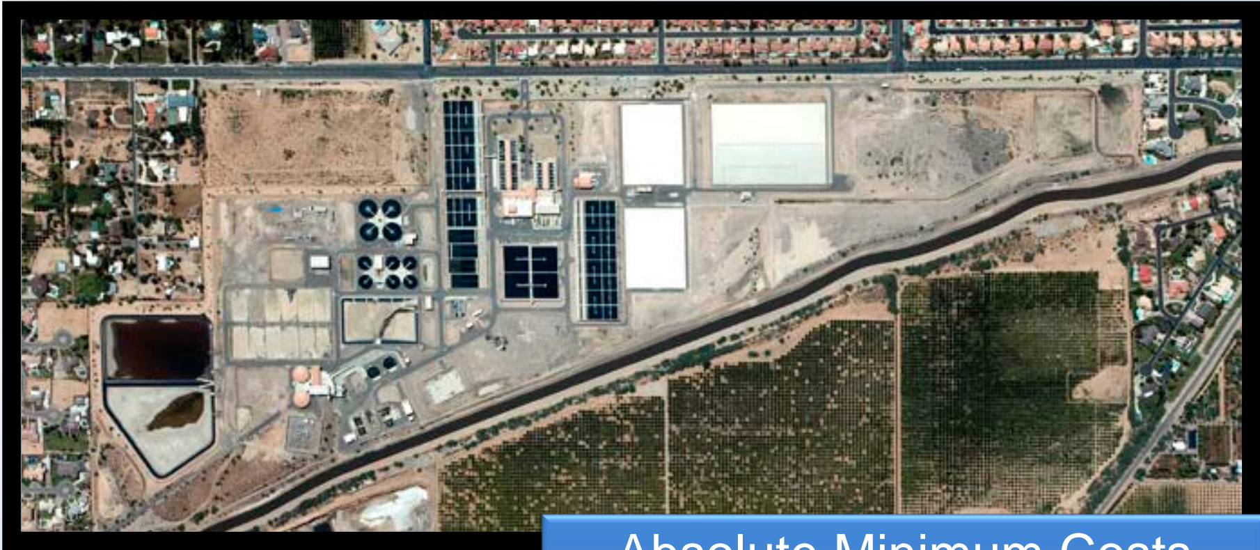
Val Vista Water Treatment Plant
