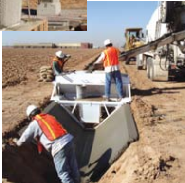
Construction of a relocated irrigation ditch
