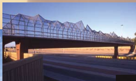
This bridge, by artist Laurie Lundquist, designed with a galvanized chain link safety cage, approximates the jagged profile of the mountains to the south.
