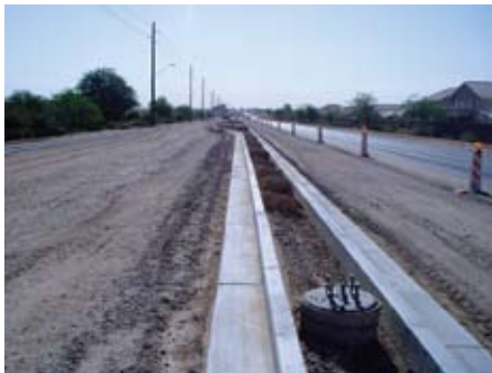
Progress continues on the widening of Van Buren Street.
