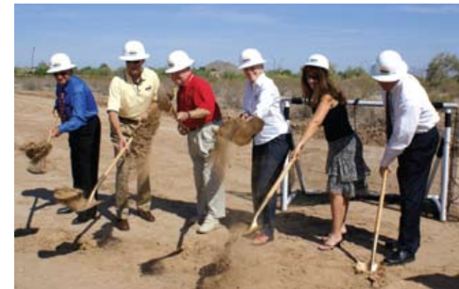
Councilmember Frank Cavalier, Mayor Jim Cavanaugh, Councilmembers Dick Sousa, Georgia Lord, Joanne Osborne and Interim City Manager Brian Dalke break ground at the site of the new City park.
