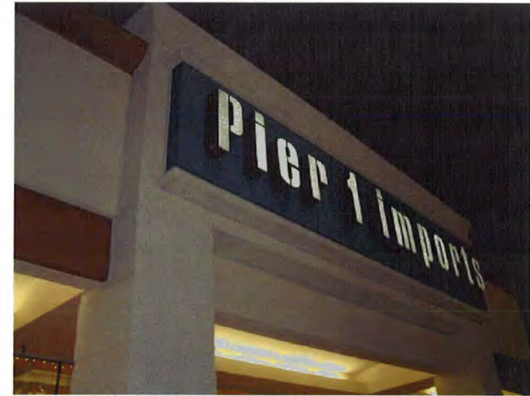
Individual plex faced letters mounted to front of metal cabinet. Cabinet is incorporated into architectural detailing.
