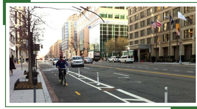
Protected bicycle lanes use physical barriers to create safer facilities for users.
