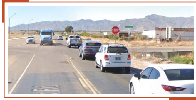
Camelback Road (looking east towards the Loop 303) is planned for widening to four lanes (see Project S5 below).
