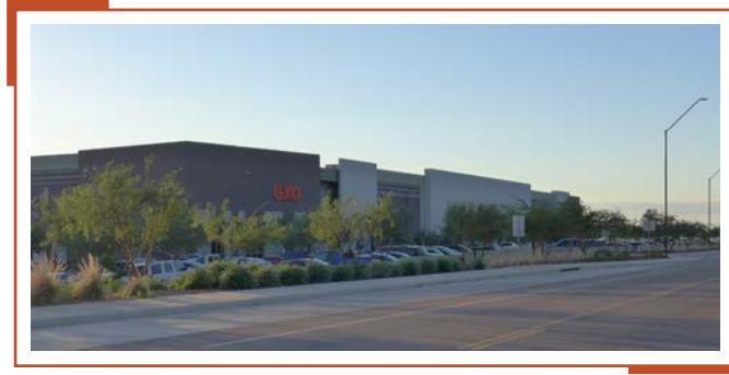
Sections of Citrus Road in north Goodyear have been improved by development.
