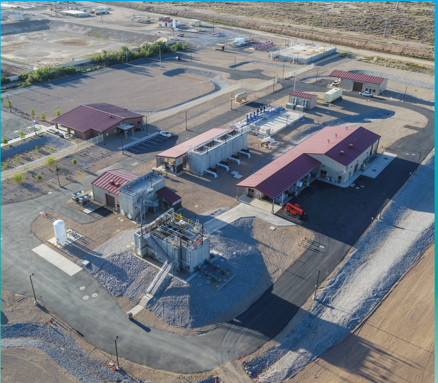
Pictured above is the city of Goodyear's Surface Water Treatment Plant which went on-line at the end of 2021.
